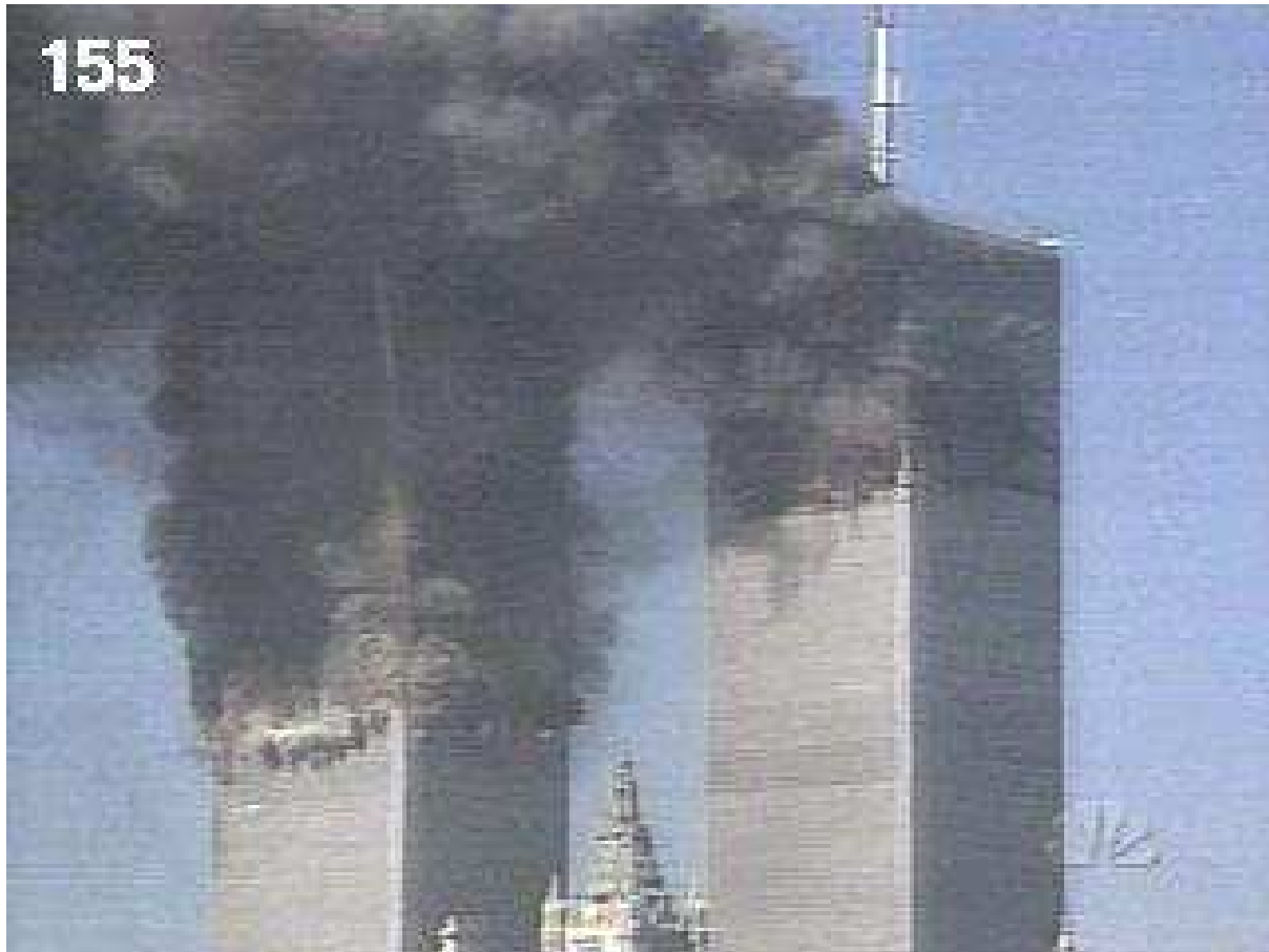
Figure 2: Towers 1.5 s later, in which the South Tower now shows substantial rapidly-moving horizontal material travelling roughly 40 mph outside of the 77th floor from which they were ejected, which was 2 floors below the lowest floor on fire.[NBC, 2001] Note the sudden leaning of the top of the South Tower at about 9^\circ , which shows no evidence of being produced by the fire. This and a subsequent horizontal ejection at floors just below this of rapidly-moving white material form the white clouds that continually develop, while the top smoke-filled segment has just started collapsing, producing the gray clouds on the right-hand side of it.
