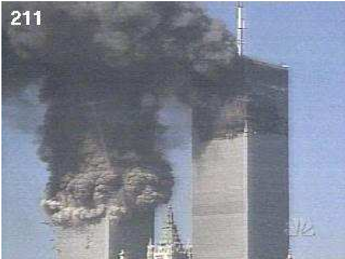
Figure 5: Photo 0.25 s after Figure 4, in which the top segment has moved further at its base with respect to the bottom (a total of about 21 m), and in which the top of the top segment has moved down in altitude over 15 m more. [NBC, 2001] The latter indicates further disintegration of the segment into the gray clouds near the bottom, which have grown substantially in size.
