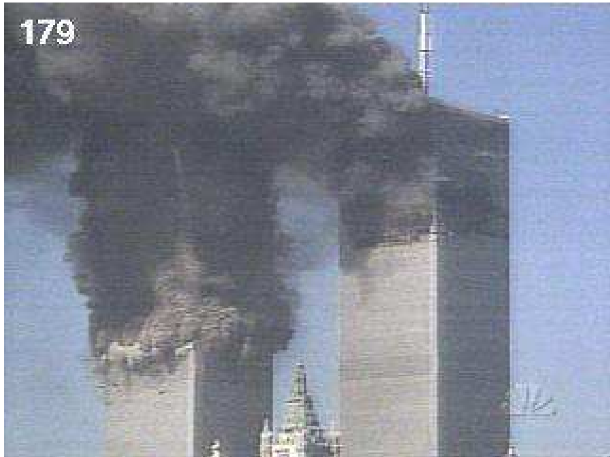
Figure 3: South tower 0.75 s after Figure 2 in which gray clouds coming from the lower part of the top segment have quickly grown to a large size, at the same time at which the top of the top segment has moved down in height. The bottom segment has not moved, but the top segment is disintegrating near its bottom. [NBC, 2001]
