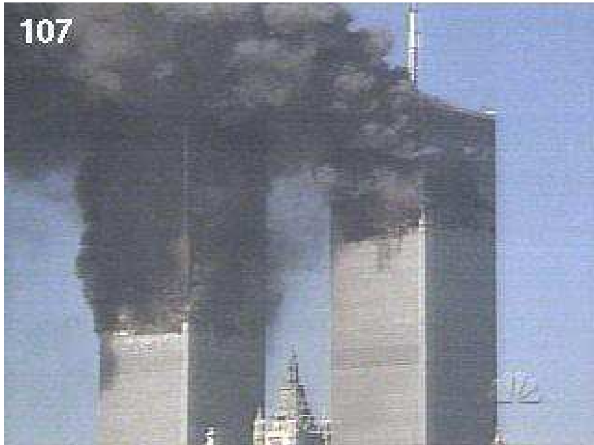
Figure 1: South tower (on the left-hand side) 56 minutes after a jet collides with floors 78 through 83.[NBC, 2001] A subtle whitening of the floor just below and at the bottom of the fire zone gives a clue of something about to happen in this distant view of the towers.
