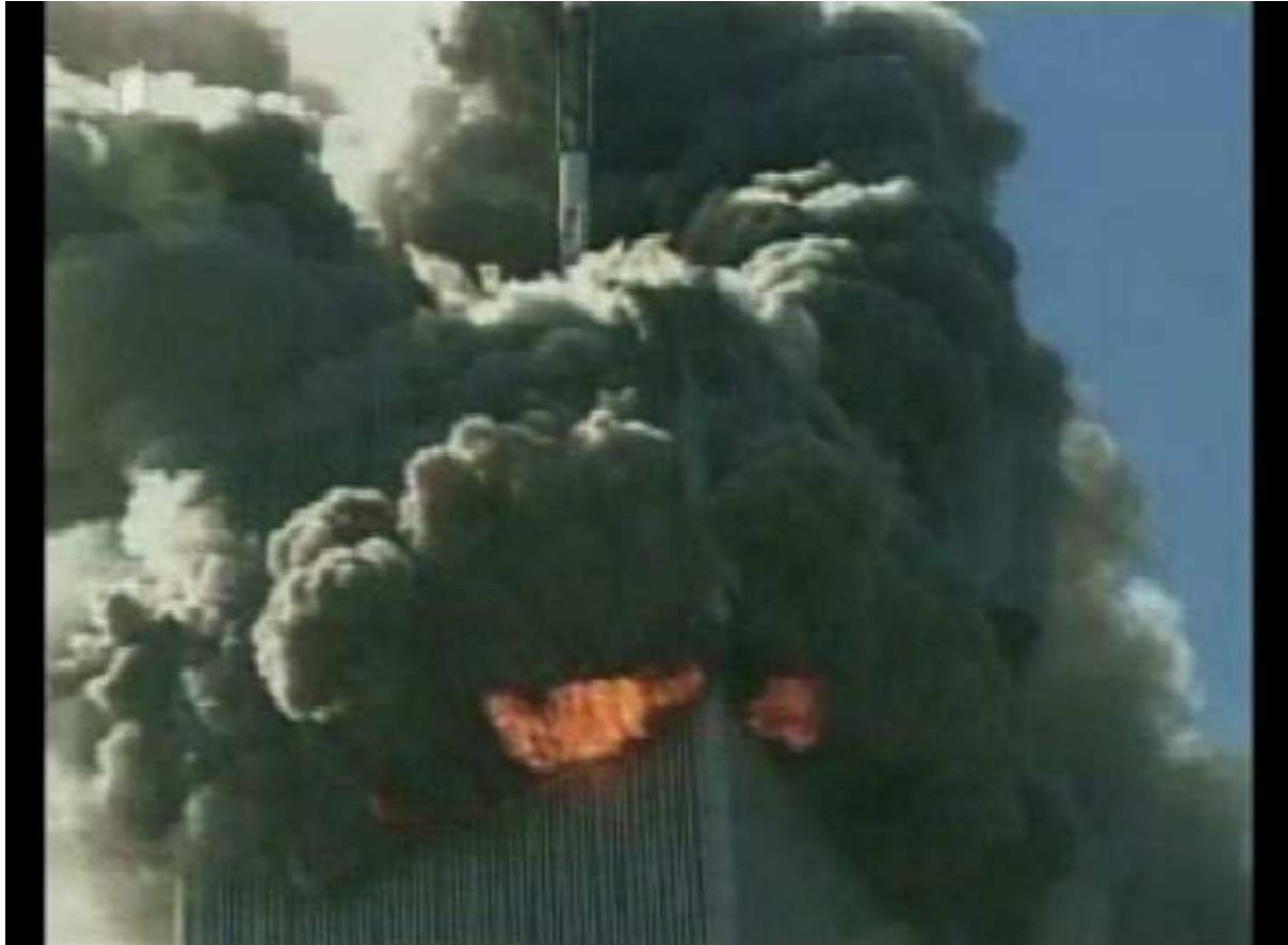
Figure 4: Heavy smoke and unusual flame emissions rapidly coming roughly horizontally out the side of the North Tower's top at velocities around 30 ft/s at the initiation of the collapse of the building, which is 0.75 s after Figure 2 [7]. Note also the antenna at the top center of the building is undergoing toppling from its position in Figure 2, implying the center of the building has a significant horizontal motion, whereas the building has not started "crushing-down". These facts are not discussed in the NIST Final Report on the collapse of the Towers.[2]
