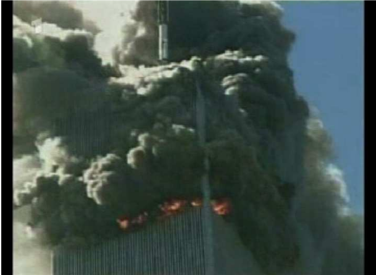
Figure 2: Perspective from North side at very initial start of collapse of the North Tower, with dust and smoke clouds very rapidly spreading out nearly horizontally, and flames at the edge of the building beginning to emerge outside the building.[7] The fire had been burning internally and steadily for 1.45 hours before this sudden eruption.
