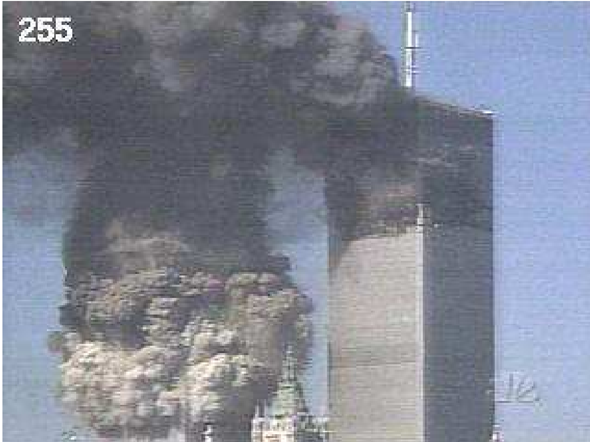
Figure 3: View of the South Tower (left-hand side) collapse just over 3 s after Figure 1, in which the top of the top segment of the Tower is collapsing below the bottom smoke line of the North Tower (right-hand side).[6] Over 50% of the top segment has collapsed and disintegrated at the bottom of that top segment, with the pulverized concrete coming out in the expanding gray clouds, while never moving down to or below the level of collapse initiation (near the top of the white clouds). The top of the top segment has dropped almost 200 ft in the under 3 s since it started dropping, suggesting a force in addition to gravity is causing it to drop. The lower segment is just starting to collapse at its very top, with pulverized concrete going into the white clouds. Nothing like a "crush-up" phase occurs for this top segment, since it never follows the bottom segment down to the ground, and collapses before the "crush-down" phase.
