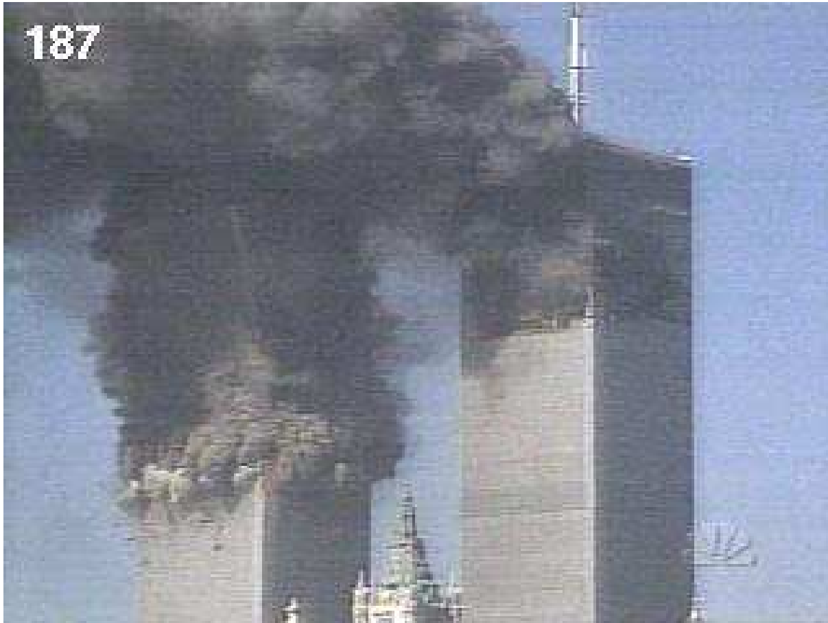
Figure 5: View of the South Tower at 9:59 AM in its collapse about 0.7 s after Figure 1, right at the beginning of forces starting to separate the top part and the lower part of the tower at its edge [6].
