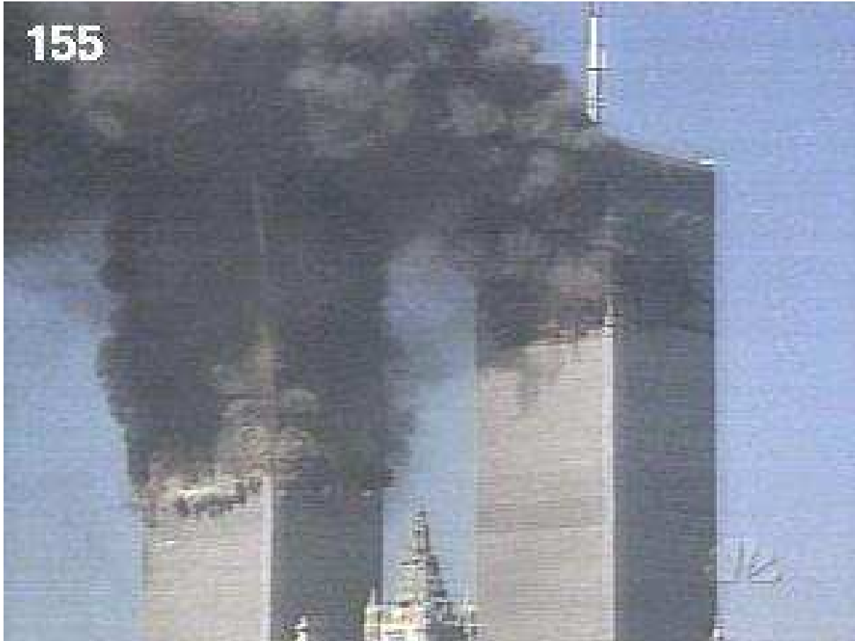
Figure 1: South tower (on the left-hand side) 56 minutes after a jet collides with floors 79 through 85, in which the rapidly-moving horizontal bursts of material travel roughly 40 mph outside of the 77-78th floors from which they were ejected, which was 1-2 floors below that lowest floor on fire [6]. There is clearly no fire in the ejected material. Fires did not produce this horizontal ejection, and the source of that momentum in the horizontal direction is not accounted for in all the NIST Committee studies. This and a subsequent horizontal ejection at nearby floors (shown in Figure 6) of rapidly-moving white material appears to form the white clouds like those in Figure 3, while the top smoke-filled segment starts rapidly collapsing moments later, producing the gray clouds like those in Figure 3. Note that the sudden leaning of the top segment of the Tower at close to 9^\circ , which also does not show any evidence of being produced by the fires.
